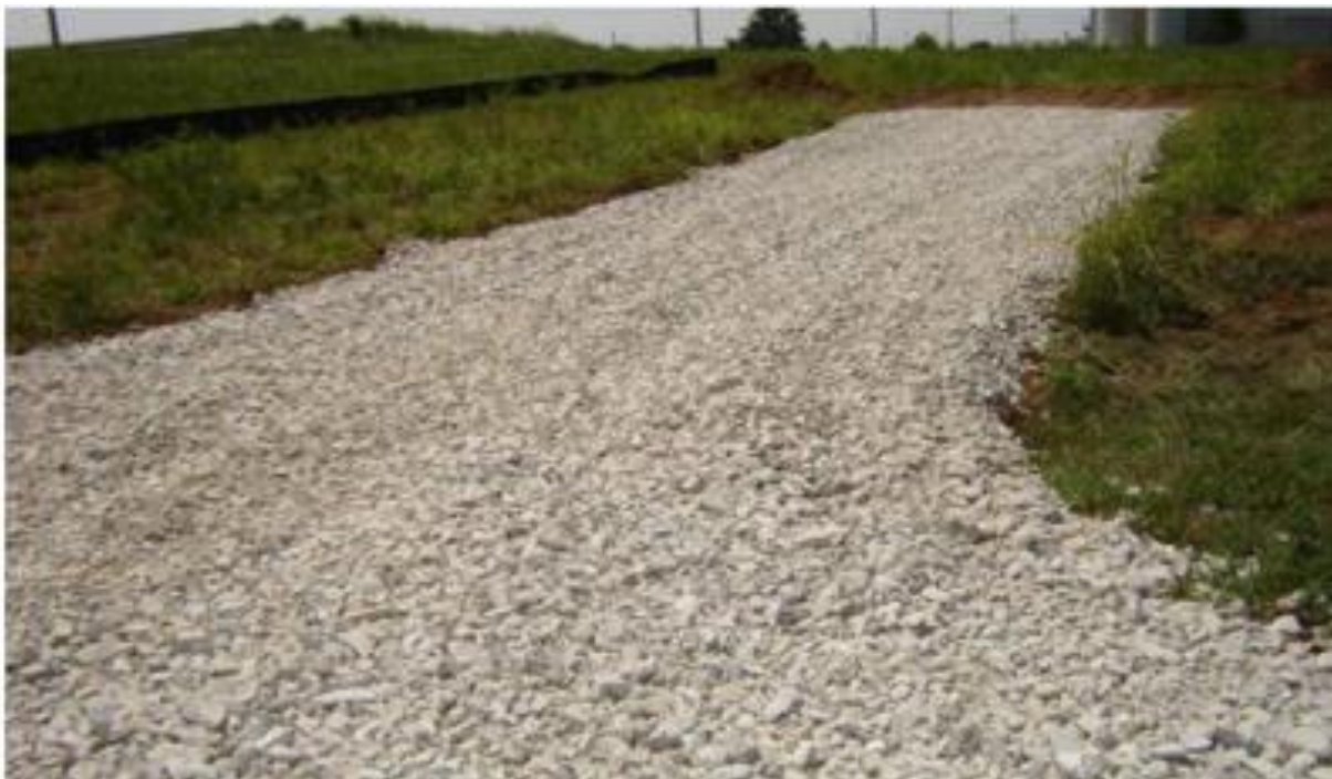
Plate 5: Temporary access track
